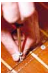
Sole boards are screwed down to keep them in situ
