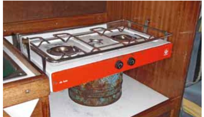
Not a recommended way of setting up your galley stove!
